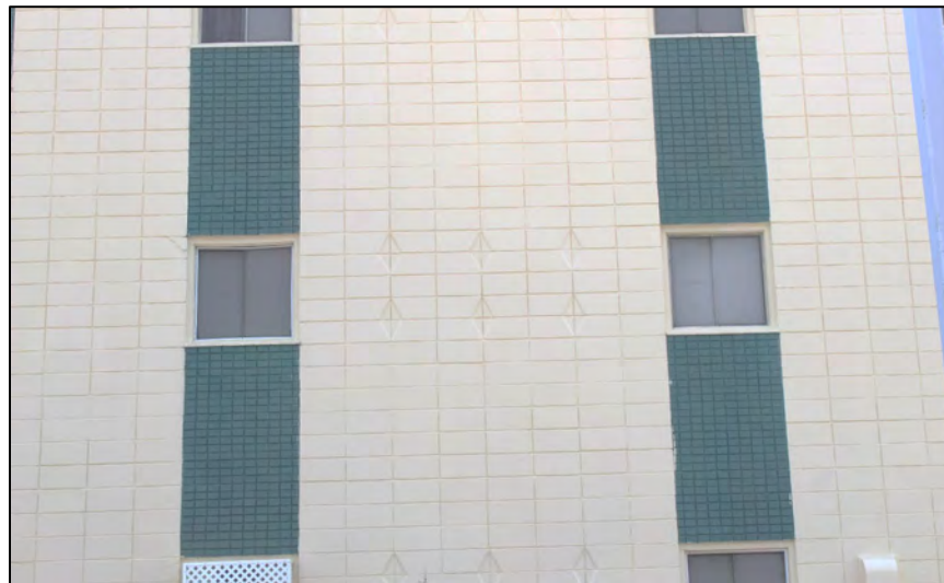
North side elevation masonry detail. September 2021.
