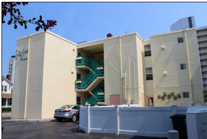
Rear elevation. September 2021.
