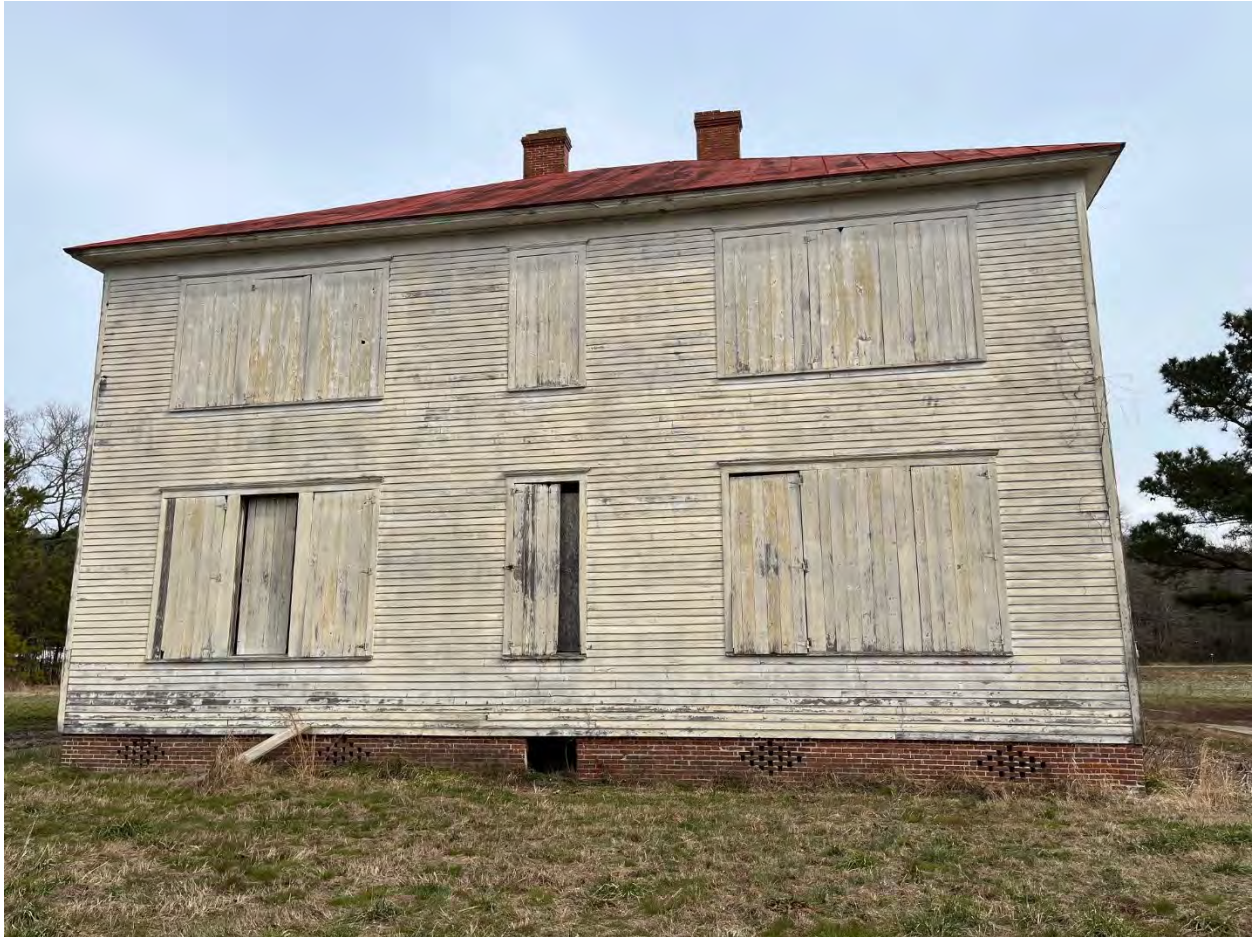
Rear (west side) of building Photographer Marian Veney Ashton
