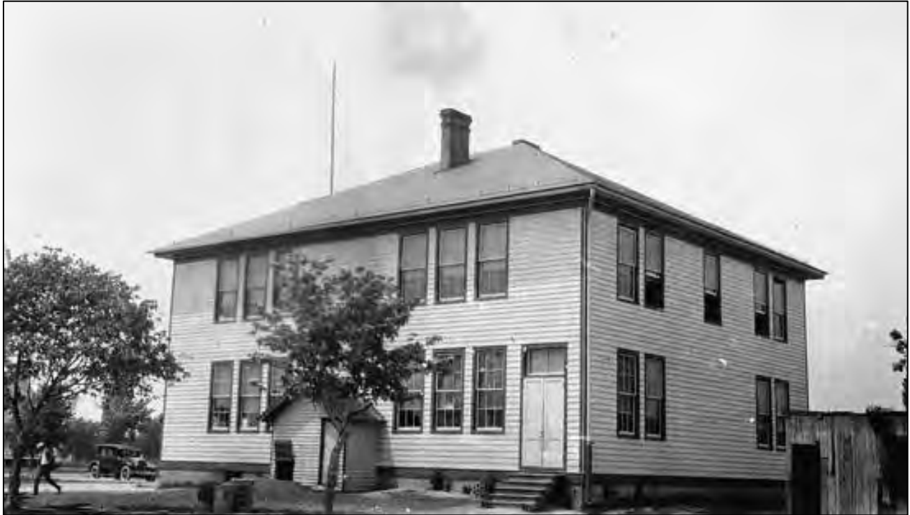
Rear [West] and Left Side [North] of Reedville School, no date. (Source: Virginia. Department of Education. Division of School Buildings. Photographs of Public Schools, 1900-1963. Accession 31032, State Records Collection, Library of Virginia. Available online at Reedville, Northumberland Co. (virginiamemory.com) ).
