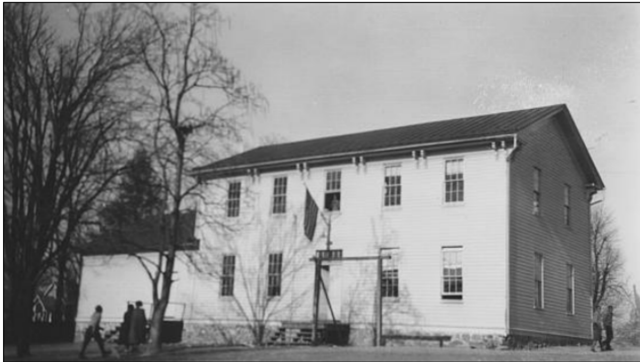
Figure 1. Ca. 1938 Photo of Union Street School. The c. 1930 addition is at left.
