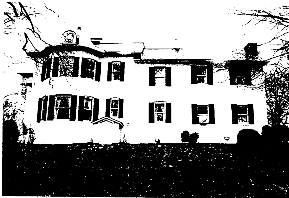
Plate 54 (top): Bel Air, west elevation, car/carrriage port, view towards east (PAV) Plate 55 (bottom): Bel Air, east elevation, view towards west (PAV)
