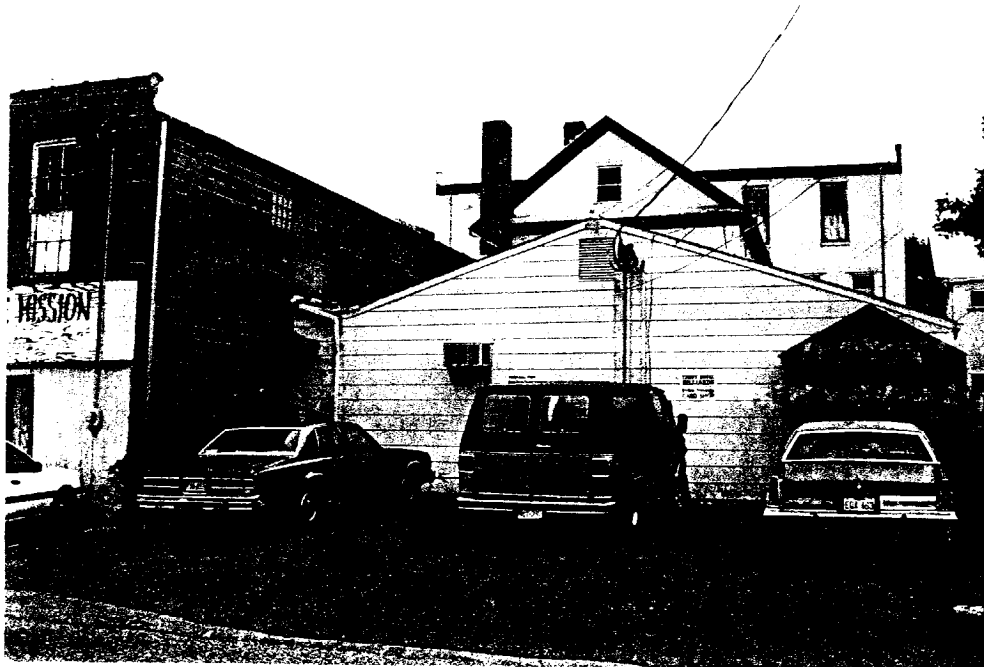
Plate 182 (top): Stickley Building (VDHR 112-0040), 21-23 South Royal Avenue, primary elevation, view towards west (Neville)
