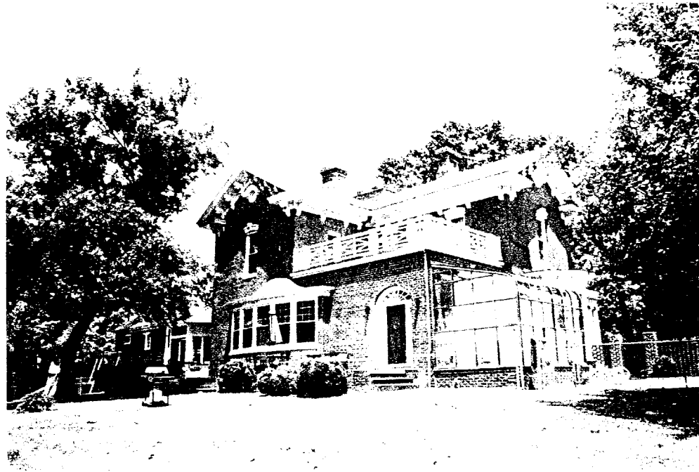
Plate 77 (top): Druid Hill (VDHR 112-0059), 1 Druid Hill Lane. primary elevation, view towards west (PAV)
